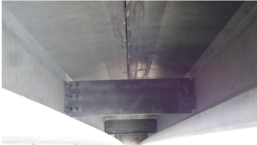
**Figure 3: Diaphragm Connecting Girders of the Bridge**
