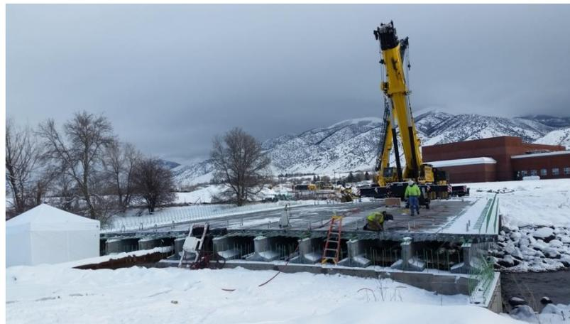
**Figure 2: Girder Placement during Construction (Ira Tibbits, personal communication, Oct. 18, 2016)**
