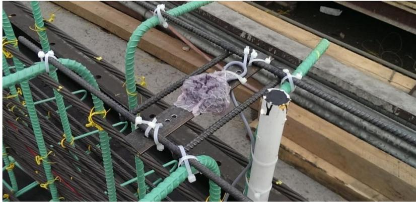
**Figure 15: Embedded Accelerometers during Construction**
