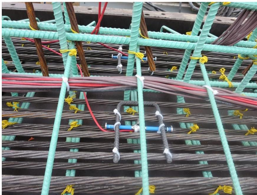
**Figure 13: Strain Gauge placed in the Web**
