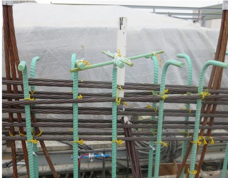
**Figure 14: Thermocouple Placement during Construction**
