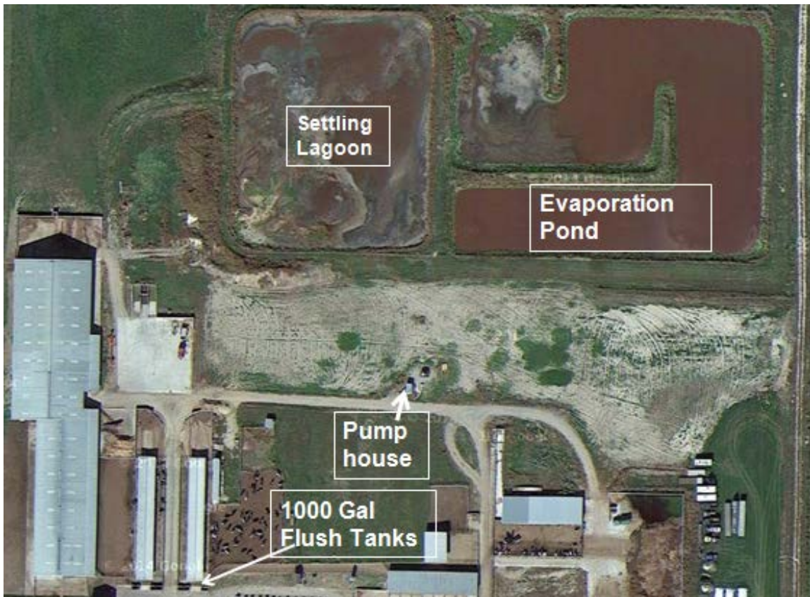
Fig. 1 Caine Dairy aerial photo. Waste management system is highlighted within the figure.
