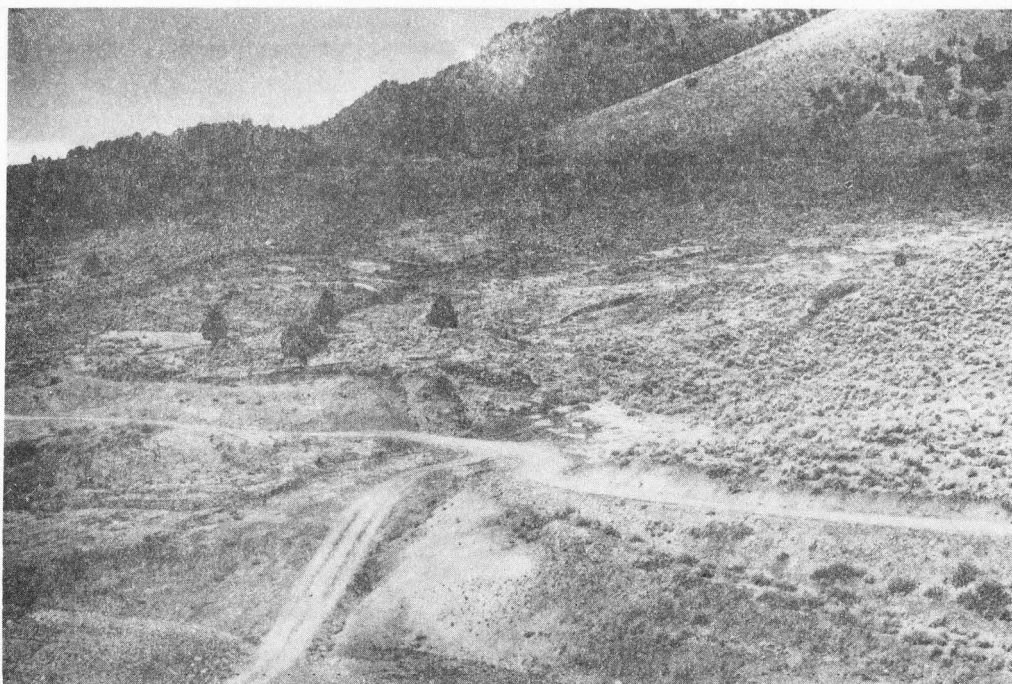
Plate 38. Closer view of landslide mass on the edge of Porcupine Reservoir.
