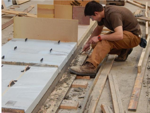
Figure 3-19 Freshly removed first layer of formwork. Scraping the hardened paste off of the concrete form base.
