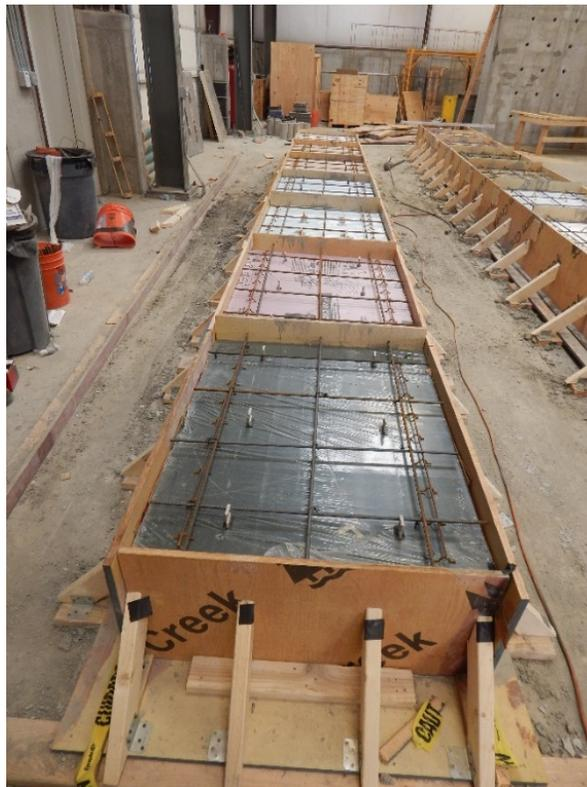
Figure 3-22 The highest set of forms is in place, ready to pour the last concrete wythe.
