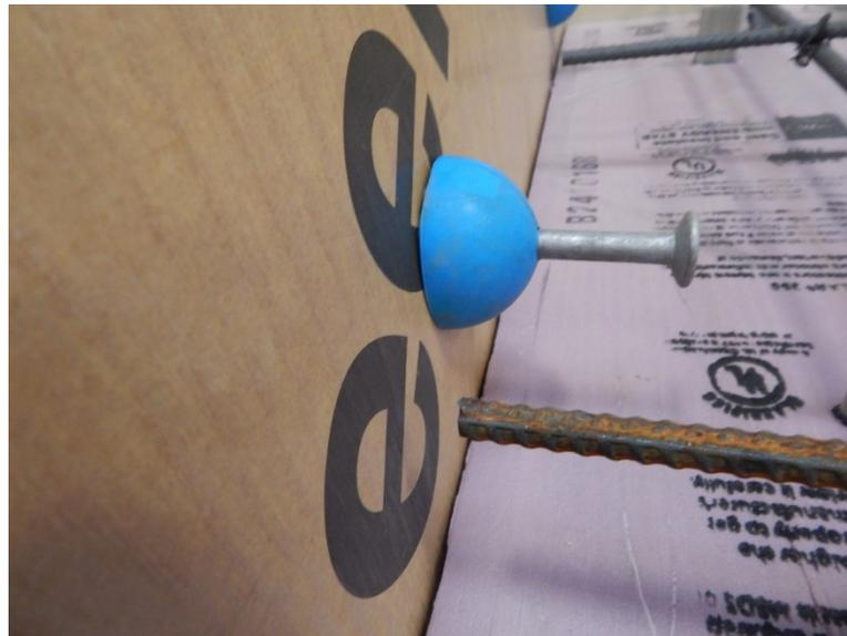
Figure 3-14 Pick points attached to divider and centered within the middle wythe.
