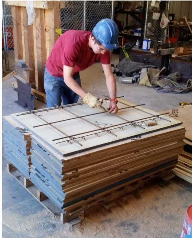
Figure 3-13 Tying rebar prior to inserting it in the formwork
