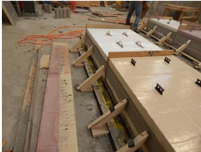
Figure 3-21 Formwork removed after concrete for the second wythe is allowed to cure.
