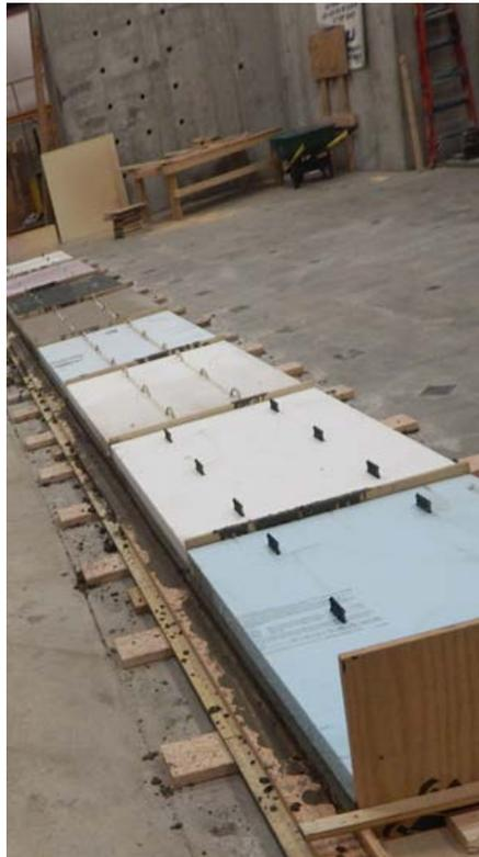
Figure 3-18 An example of a completed first layer. Concrete has been poured and foam and connectors have been put in place.
