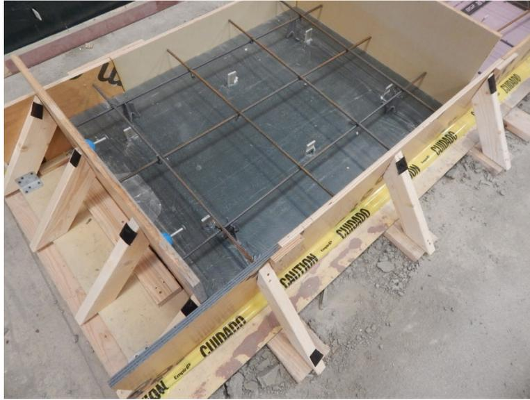
Figure 3-20 Prepared second wythe. Rebar, pick points, and form work are all in place.
