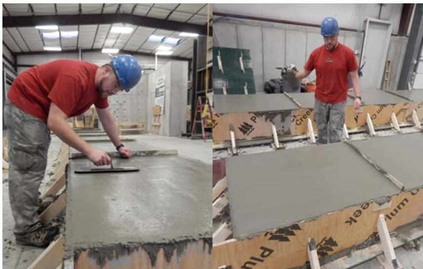
Figure 3-23 Taking special care to put a finished surface on the final wythe of the concrete.
