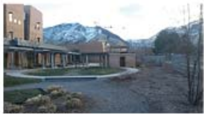
PERGOLA #1 (INSUFFICIENT SHADE STRUCTURE)
