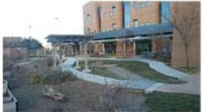
PERGOLA #2 (INSUFFICIENT SHADE STRUCTURE)
