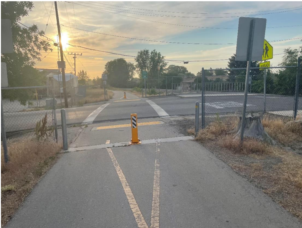
Figure 4-11. Trail intersection treatment with collapsible bollards.
