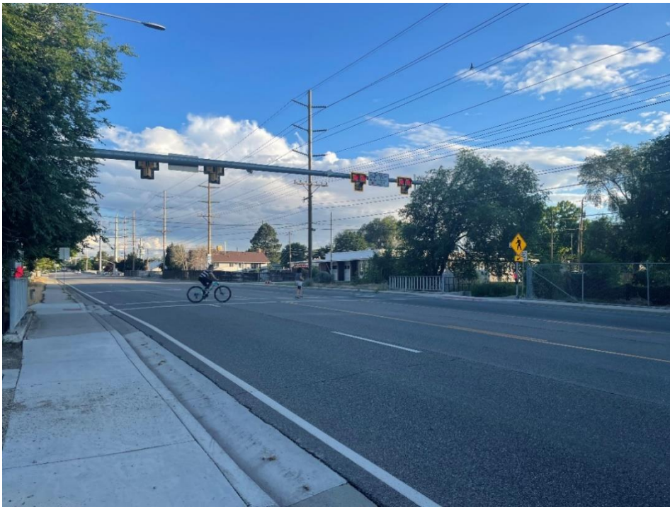
Figure 4-10. Pedestrian hybrid beacon at canal trail intersection.
