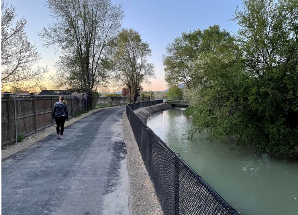
Figure 4-2. East Jordan Canal Trail with fencing between the canal and trail.
