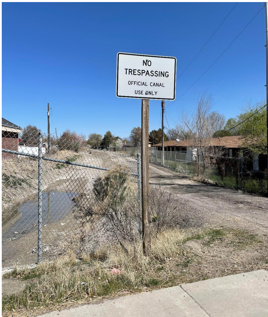
Figure 2-1. No trespassing signage at canal corridor entrance.
