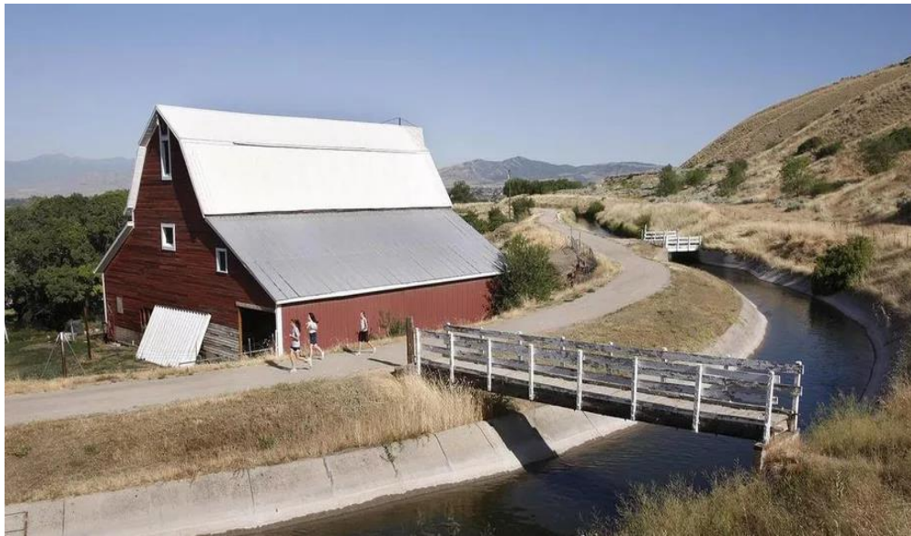
Figure 4-14. Murdock Canal prior to enclosure. (Johnson, 2013).
