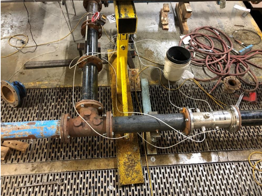
Figure 8. UVT with taps at positions 1 and 2 installed 5D on the through leg of a round cornered tee junction.
