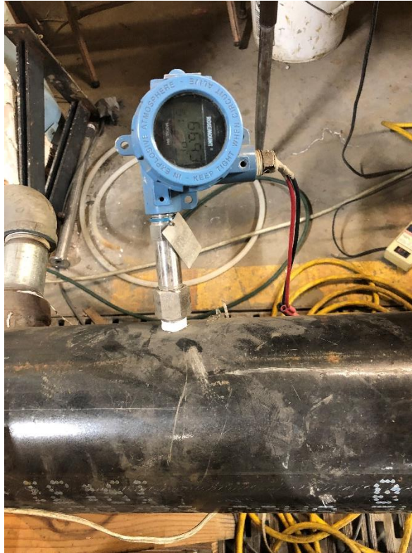
Figure 11. Temperature probe installed on the test pipeline.
