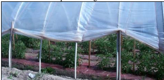
Figure 2. Side ventilation of a tomato high tunnel.
