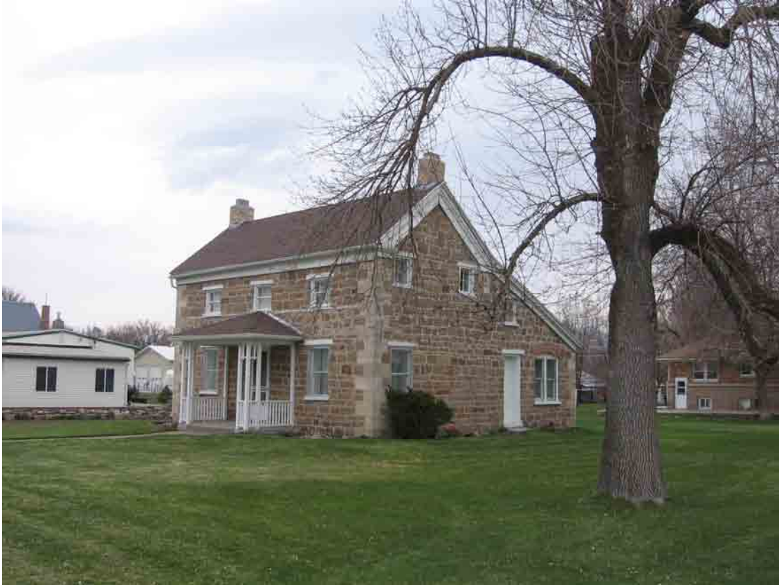
Figure 4: Zial Riggs house, built ca. 1861. Picture by author 2008.
