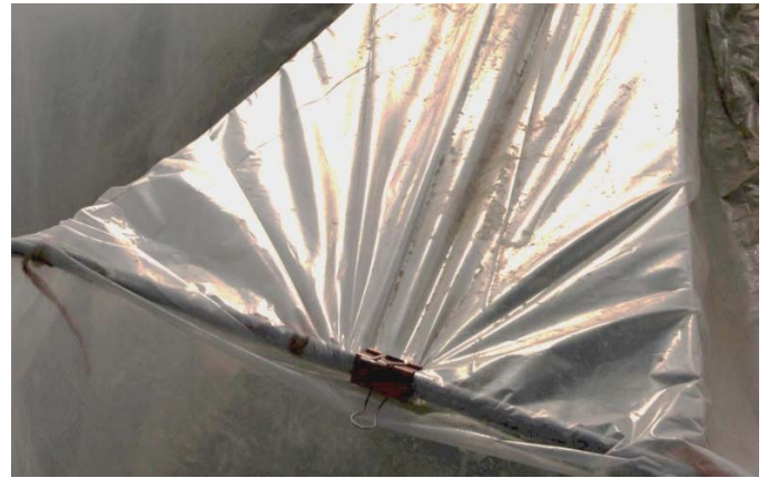
Image 7. Binder clip securing plastic to conduit frame.
