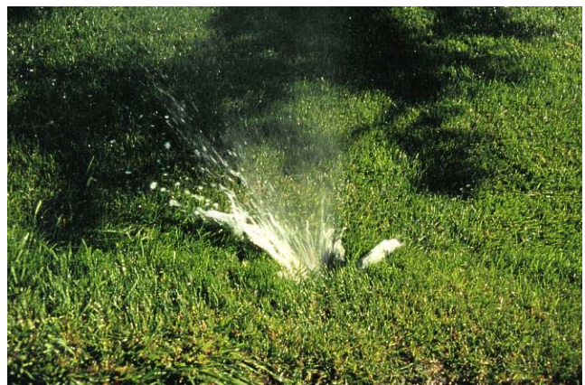
Figure 6. Sunken sprinkler head and distorted spray pattern.
