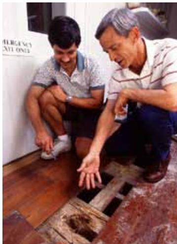
Fig. 10. Subterranean termites can shred solid wood beams.<sup>4</sup>
