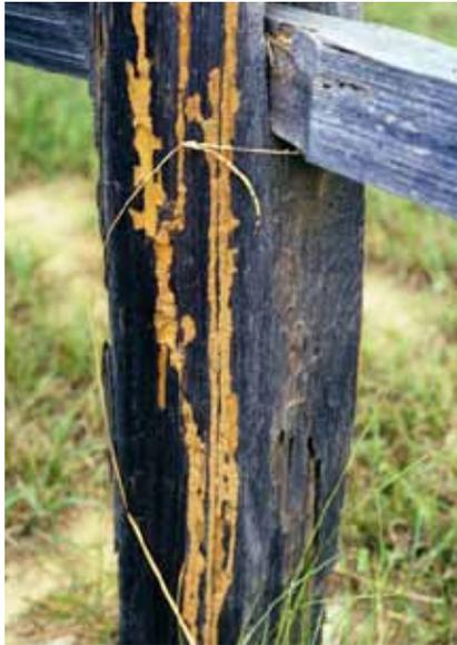
Fig. 7. Eastern subterranean termite mud tubes on a post.<sup>6</sup>
