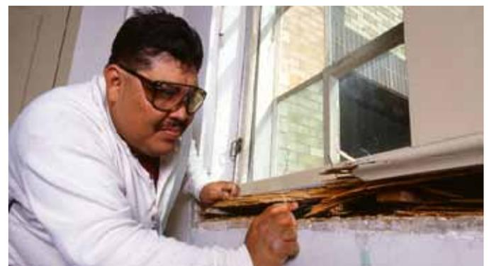
Fig. 9. Heavy subterranean termite feeding damage can cause paint to blister.<sup>4</sup>
