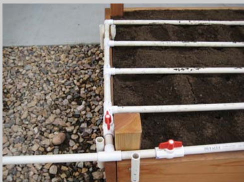
Manual valves control flow rate and assist in reducing pressure
