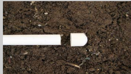
End caps are not glued for ease of cleaning the system
