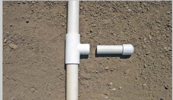
Plugs are used to eliminate watering non-irrigated rows
