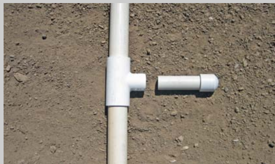
Plugs are used to eliminate watering non-irrigated rows
