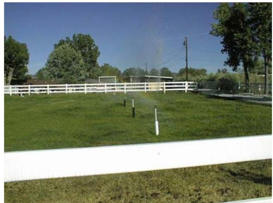
Water discharged from a sprinkler into the air should infiltrate the soil where it falls, there should be no runoff. For high uniformity of wetting, the spray patterns from adjacent sprinklers must properly overlap. Generally, in a full coverage situation, the spray from
