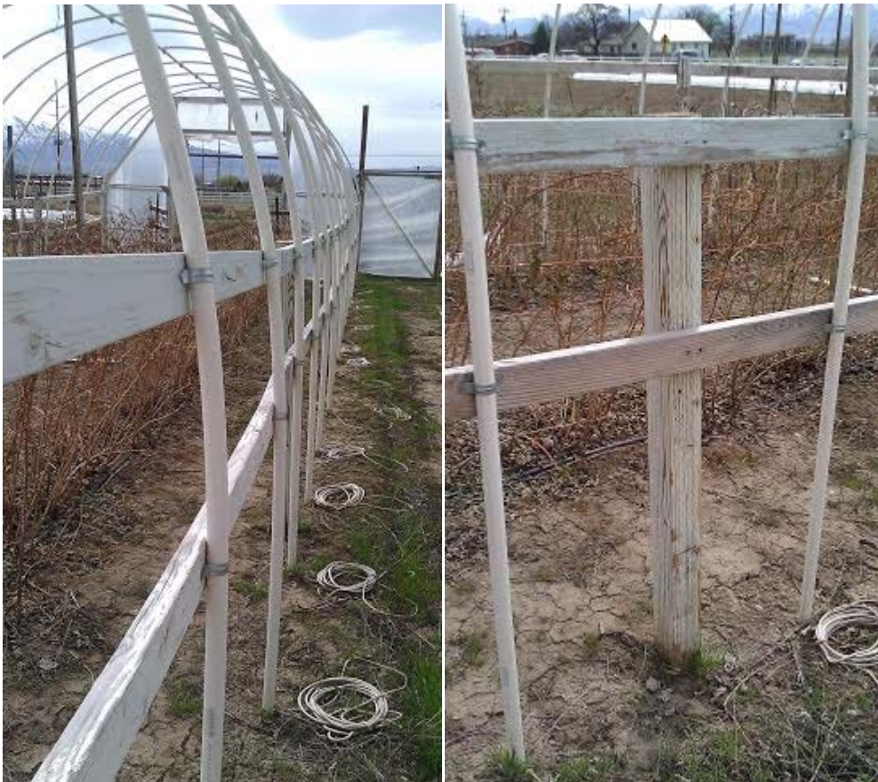
Figure 1. 2x4 side supports connected to PVC hoops and 4x4 anchor. Coils of rope attached at the base of each arch will be stretched over the tunnel to further tension the plastic.
