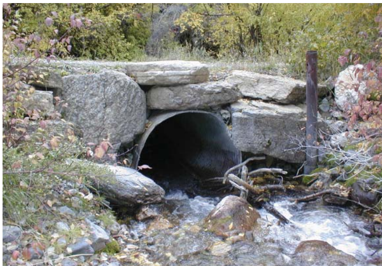
A well-constructed stream crossing will protect water quality and fish habitat for future generations.
