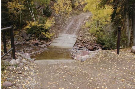
This ford on the headwaters of the Weber River has a firm rock bottom and the approaches have been hardened with concrete.
