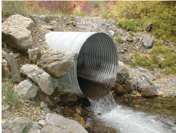
Waterfalls from culverts scour the stream bed and make fish passage difficult. Aligning the culvert with the stream gradient is the preferred practice, although rock armoring can be used here below the waterfall to reduce scouring and above the culvert to reduce road erosion.
